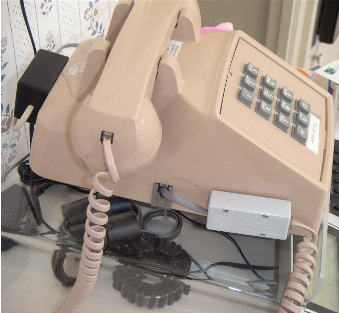
Figure 16: K-COM modular four-wire common-mode choke on the handset cord, and K-Y modular two-wire common-mode choke on the line cord, of our kitchen telephone. Also visible, through the transparent plastic telephone stand, are a home-brew 5943003801 toroidal choke on the low-voltage power cable, and a four-bead binocular-core choke on the telephone line cable, of a Caller-ID box.
